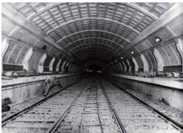
1— Works in progress of the Transversal subway, Barcelona, ca. 1920.
